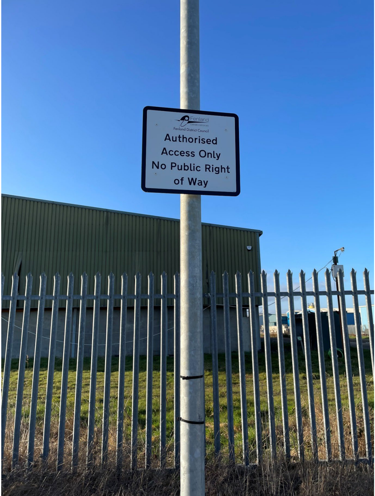
Photograph taken 23 February 2023. View west into Algores Way Waste Transfer Station, Algores Way, Wisbech
